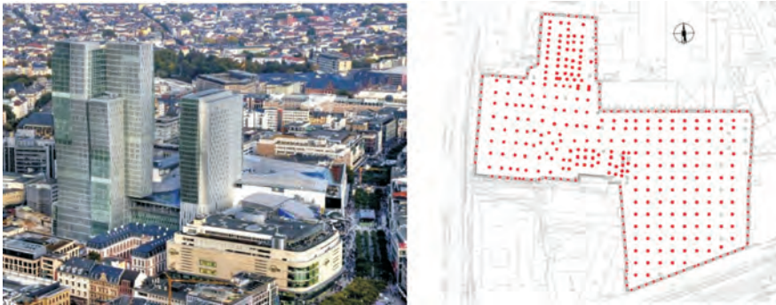
Figure 5 – Top image and layout of energy piles of PalaisQuartier, Frankfurt am Main
