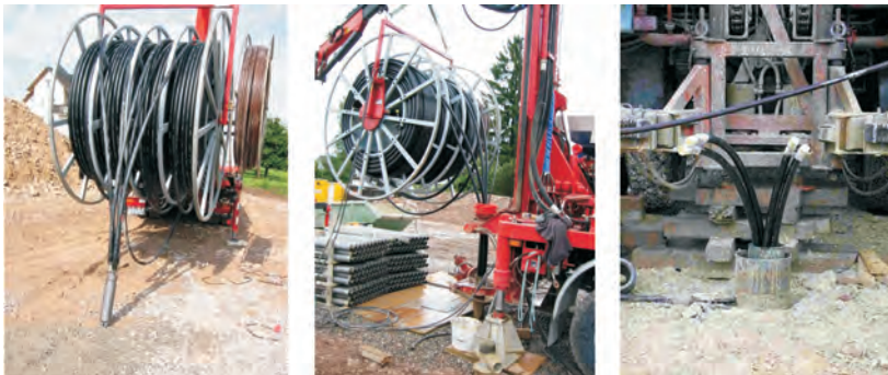
Figure 3 – Installation of Double-U-Tubes for borehole heat exchanger
